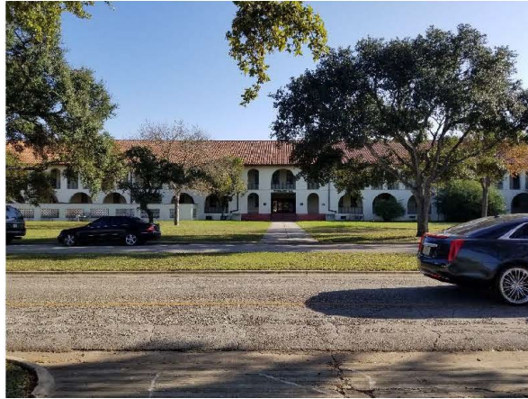
Building 399, SE of the proposed construction site
