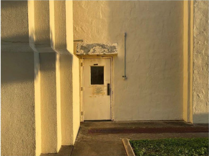
Door, NW Corner
